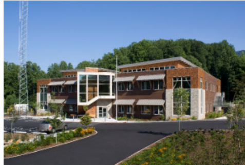
EBCI Shawn Blanton Emergency Operations Center
