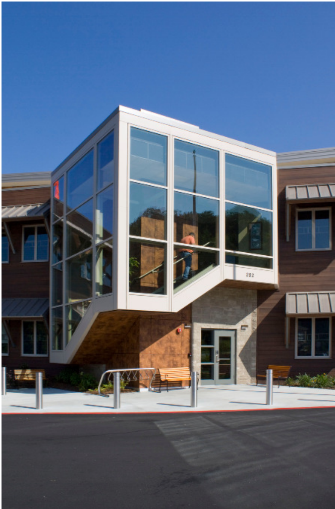
EBCI Emergency Operations Center
