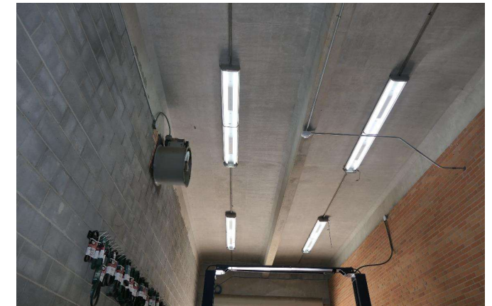
Interior ceiling at vehicle repair bay
