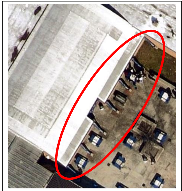
Cafeteria (7 total – all on inside courtyard side)
