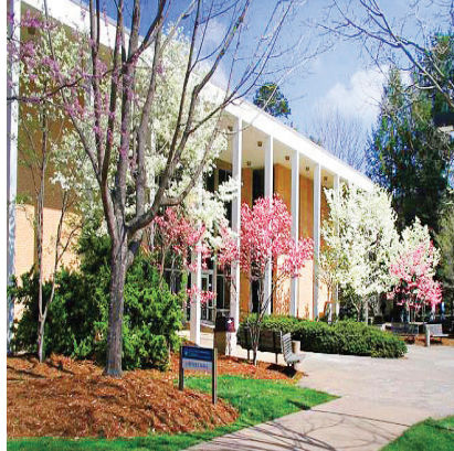
LIPINSKY HALL RENOVATION UNCA
