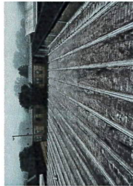
Original standing seam metal roofs
