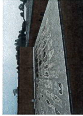
Roof covering at EC Wing in poor condition
