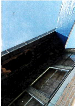
Original standing seam metal roofs
