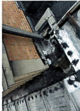
Poor drainage detailing and area of persistent water ingress
