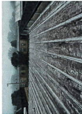
Original standing seam metal roofs
