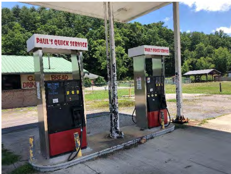
Photograph 5: View of fuel dispensers. Two suspected UST vent pipes are present adjacent to support post to canopy in center of photograph. View is to the southeast.
