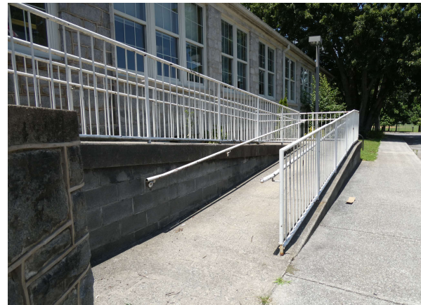
Exterior view of entrance ramp with guardrail.
