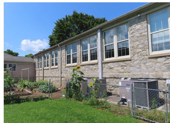
Stone faced walls and double pane aluminum and vinyl windows.
