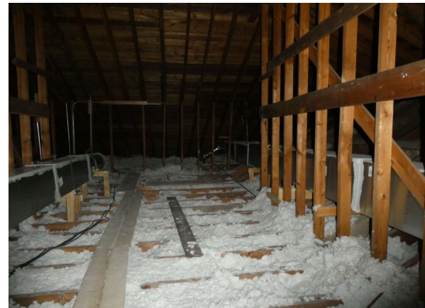
Architectural wood frame structure.
