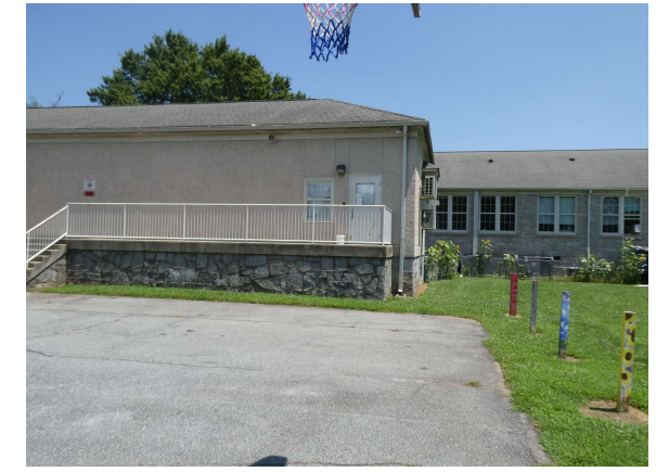
Modular unit addition with stucco exterior.
