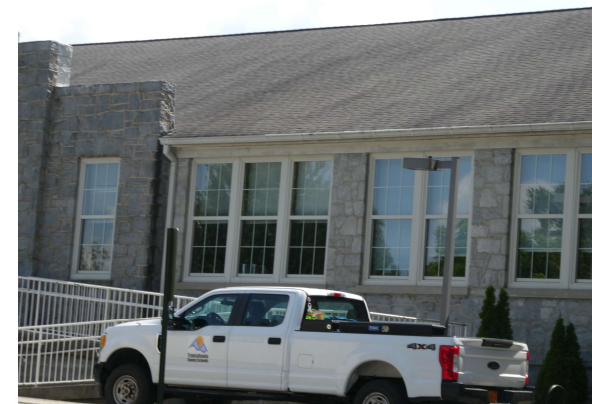
Stone face exterior and vinyl hung windows.
