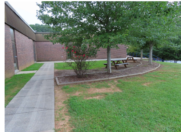
Landscaped area that holds water in heavy rain
