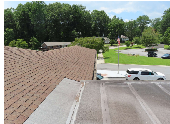
Low slope built up asphalt shingle roof
